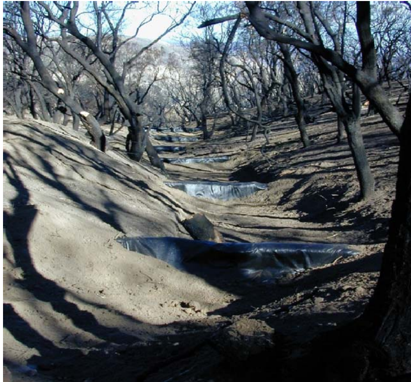
Figure 7. A series of log check dams on the Piru Fire (photo by Allen King)
