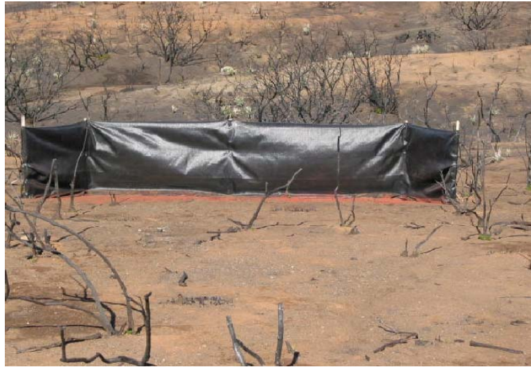
Figure 5. Silt fence for Measuring Hillslope Erosion
