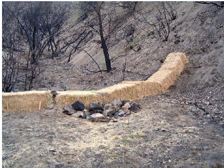
Figure 6. Straw Bale Check Dam in a Steep Channel on the Old/Grand Prix Fire (photo by Vicky Sjöberg)
