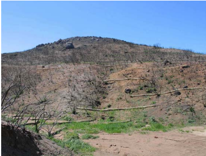
Figure 3. Fiber Rolls in an Overlapping Pattern with Spacing Inversely Proportional to Slope Angle on the Cedar Fire
