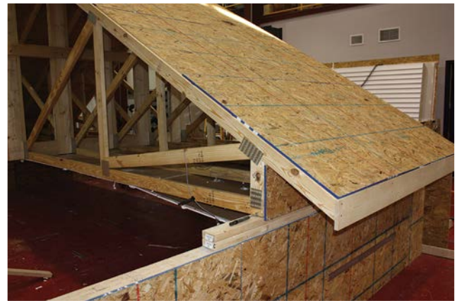
Figure 18. Truss rotation of Specimen E at failure (Truss 5).
