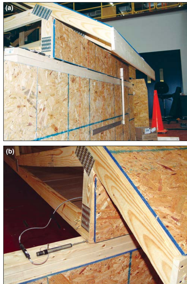
Figure 17. Comparison of rotation at Truss 5 (Specimen D): (a) before test, (b) after test.
