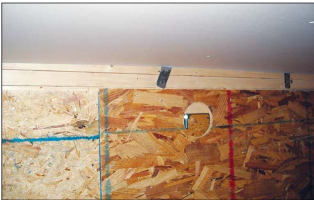
Figure 13. Rotation of hurricane clip at failure (Specimen A).
