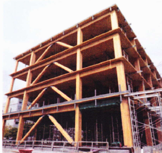
Figure 4. The Earth Science Building at the University of British Columbia under construction in British Columbia, Canada (photo courtesy of Structurlam, Penticton, BC, Canada)
