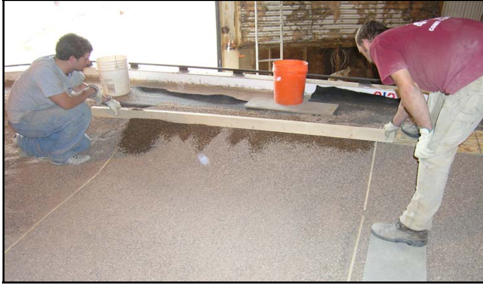
Figure 2.10: Skreeding of Rock Fill (Walker 2009)
