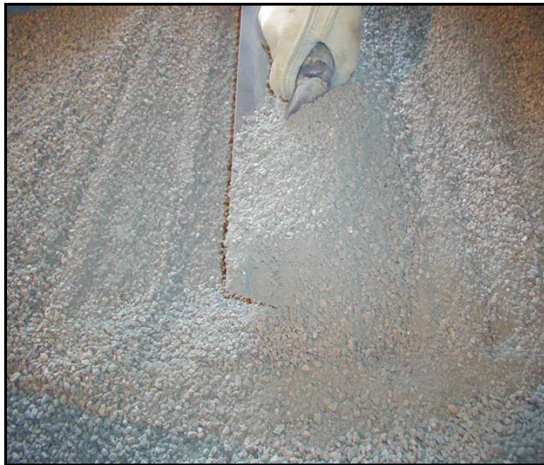
Figure 2.11: Shifting or Cutting-down Portland Cement into Gravel (Walker 2009)
