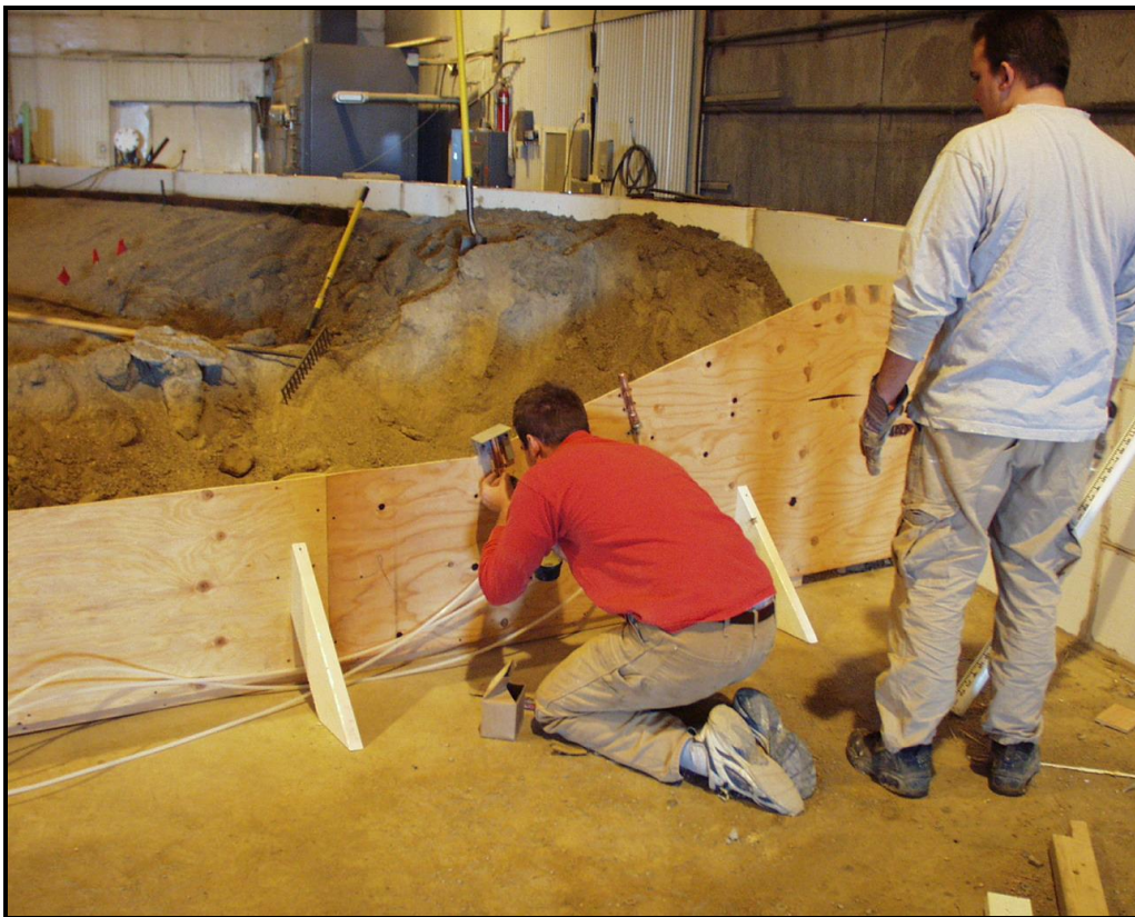
Figure A.14: Installation of Piezometer for Flow Depth Measurement
