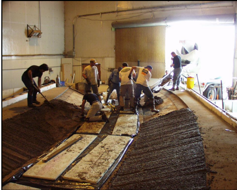
Figure A.9: Pouring of Concrete for Model Construction
