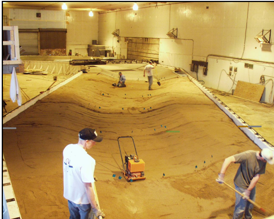
Figure A.7: Leveling of Fill Sand of the Main Channel
