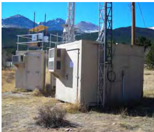
CASTNET monitoring site in Rocky Mountain National Park, Larimer County, CO (photo courtesy of U.S. EPA).
