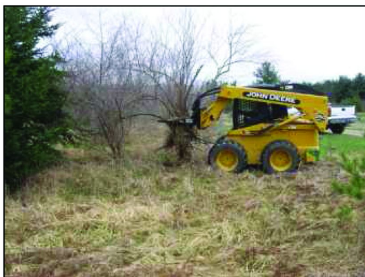
Figure 10. Grubbing machine. Image by Steven Manning, Nashville, Tennessee.
