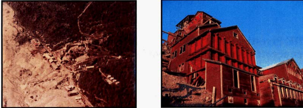
Figure 1 –Aerial view of the Kennecott Mine complex (left) and a northwest view of the Concentration Mill Building (right).
