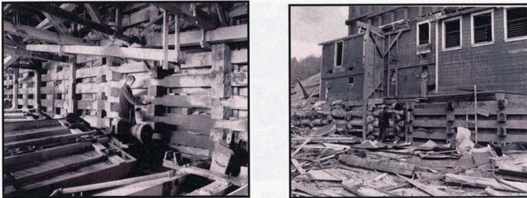
Figure 2 - Timber crib foundation wall (level 3, left) and outside (level zero, right) during the 1976 building inspection.
