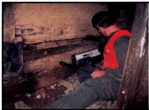
Figure 3 - Moisture content measurements being collected with an electrical-resistance-type meter.
