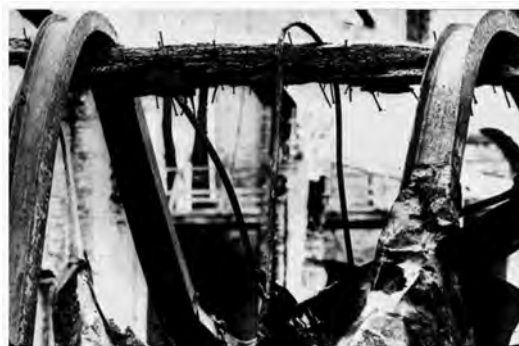
FIGURE 6.9 Wood beam survives fire in casein plant in Frankfort, NY.
