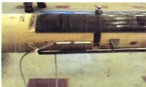
Figure 7: Example of the Type B shear failures seen in the gusset style connection
