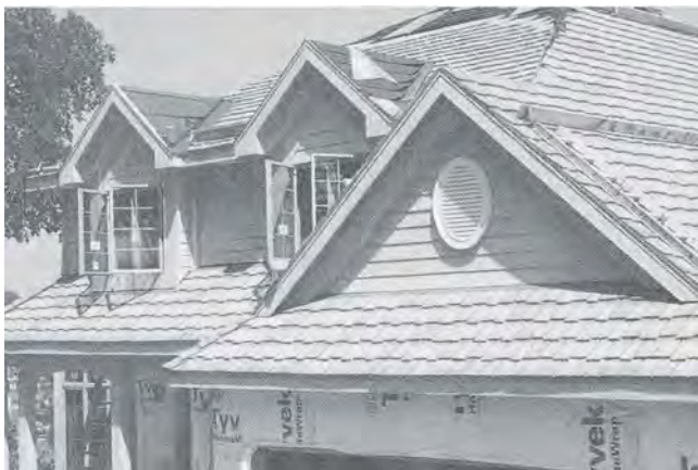
FIGURE 13.6 WPC roofing tiles.
