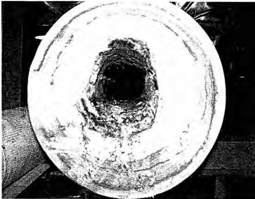
FIGURE 7.1. Calcium oxalate scale constricting flow in a pipe.
