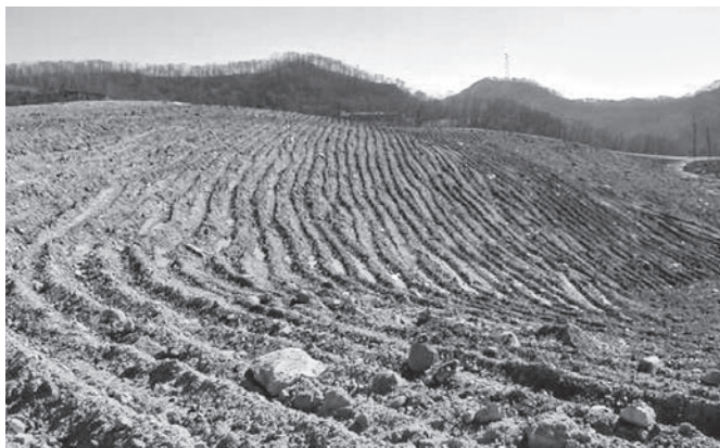
Figure 2. A single shank ripper pulled by a D11 was used on this gently sloping area to a depth of \approx 2 m on the University of Kentucky's Bent Mountain Reforestation Research Complex in Pike County, Kentucky. Surface water retained in the rips reduces runoff, erosion, and sedimentation.
