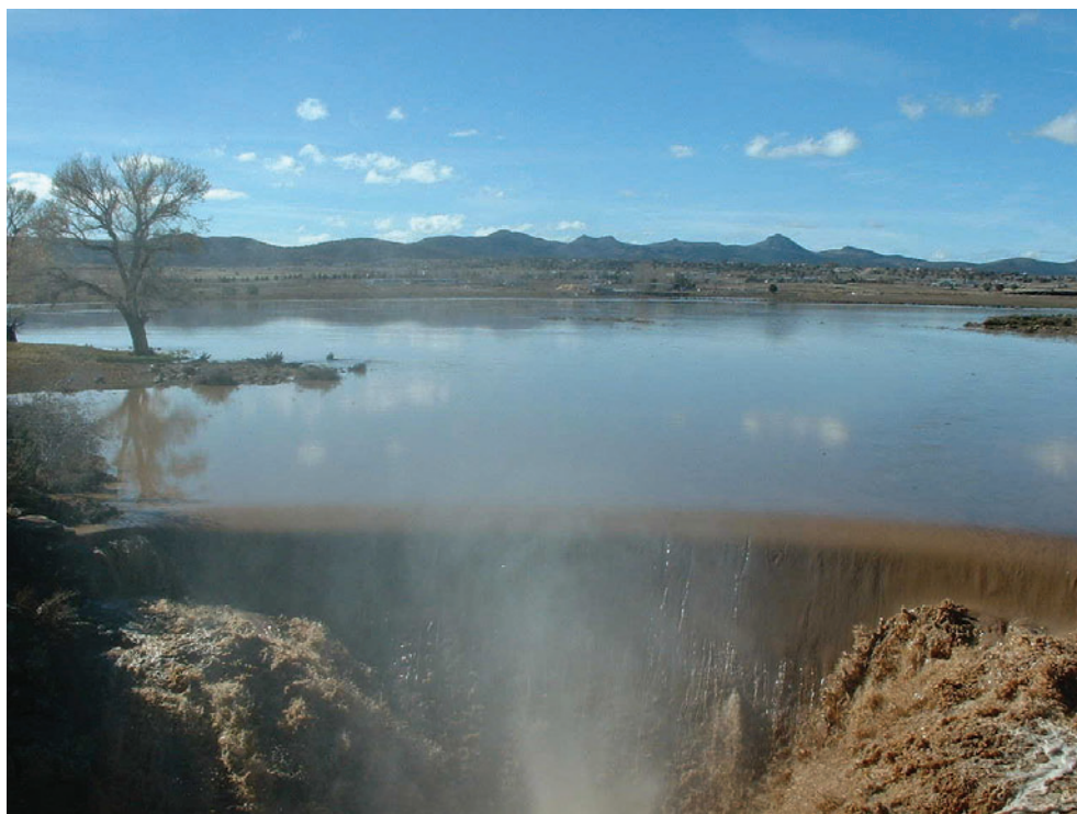
Figure 9.8— Flow over Sullivan Dam during spring runoff, 2005. (Photo by Alvin L. Medina.)
