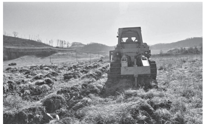
Figure 1. Single shank ripping with a D9 dozer on an abandoned surface mine site near White Oak, Tennessee.
