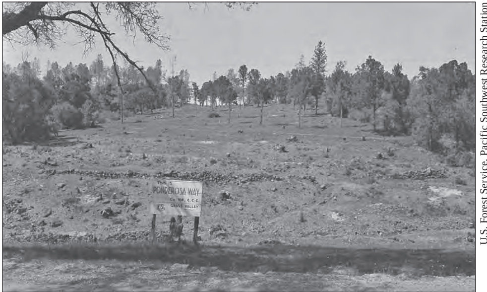
Figure 55—Ponderosa Way constructed by the Civilian Conservation Corps near Grass Valley, California, 1934.
