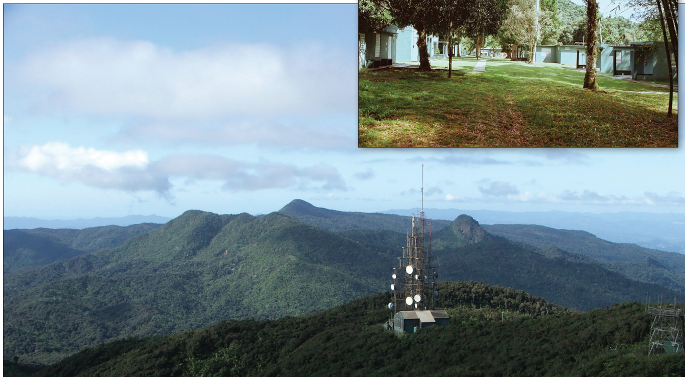
ABOVE: Built in the late 1940s and consolidated in the early 1980s, the island's major communication towers are situated at nearly 1000 m elevation along the spur road to El Yunque peak. (Photo by Iván Vicéns) ABOVE RIGHT: The Eliza Colberg girls scout camp, dedicated in 1950, has provided an outdoor training center for generations of youngsters. (Photo by Peter L. Weaver)
