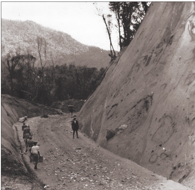
Construction of PR route 191 from Palmer to Naguabo started in 1926 and was completed in 1942. The road traversed the Luquillo Mountains and later provided access via tributary roads to the summits of El Yunque, Pico de Este, and Pico del Oeste. (Photo from IITF files)
