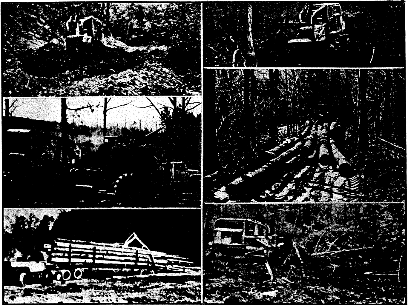
Figure 2.-Truck road construction, system move between landings, skidding, trucking, and landing construction times are computed in L-O-S-T.
