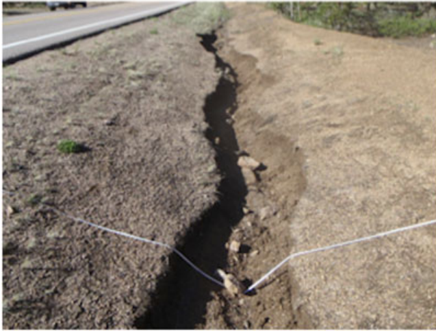
Figure 3. An incised drainage ditch associated with Pikes Peak Highway. Source: Troendle et al. , unpublished report. 2010, pp 1–34. This figure is available in colour online at wileyonlinelibrary.com/journal/espl
