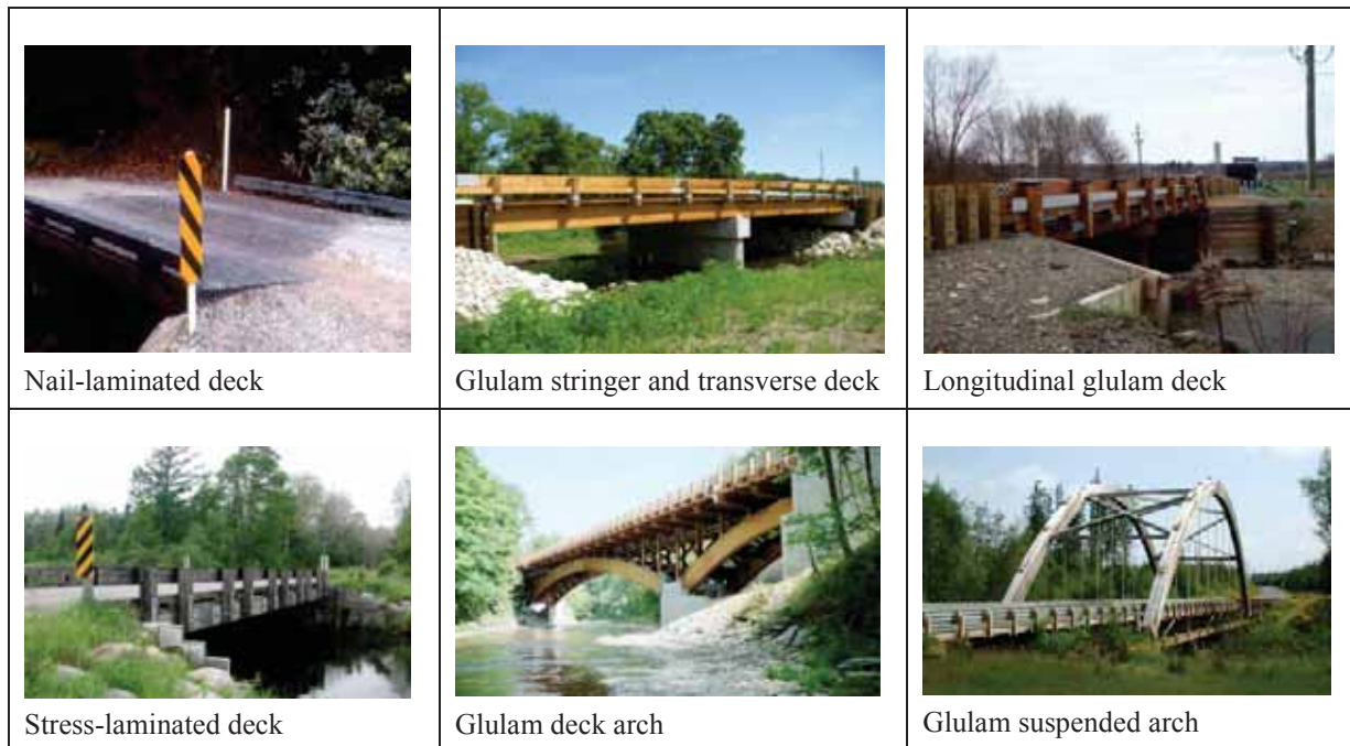
Figure 2 —Examples of various timber bridge superstructures.
