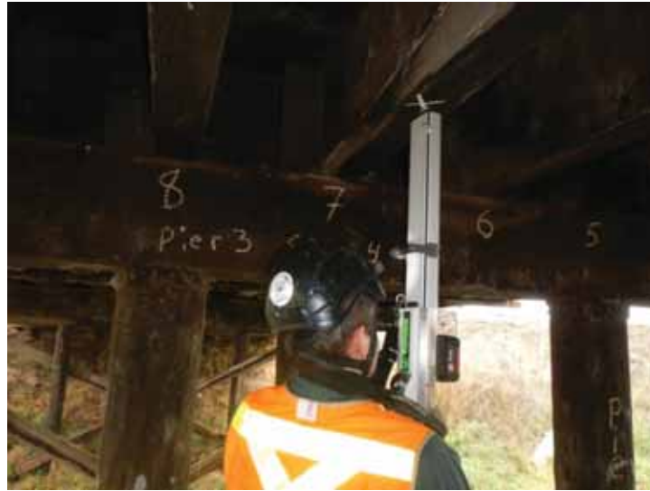
Figure 4 —Inspection of a timber bridge superstructure located in Washington using a resistance micro-drilling unit.
