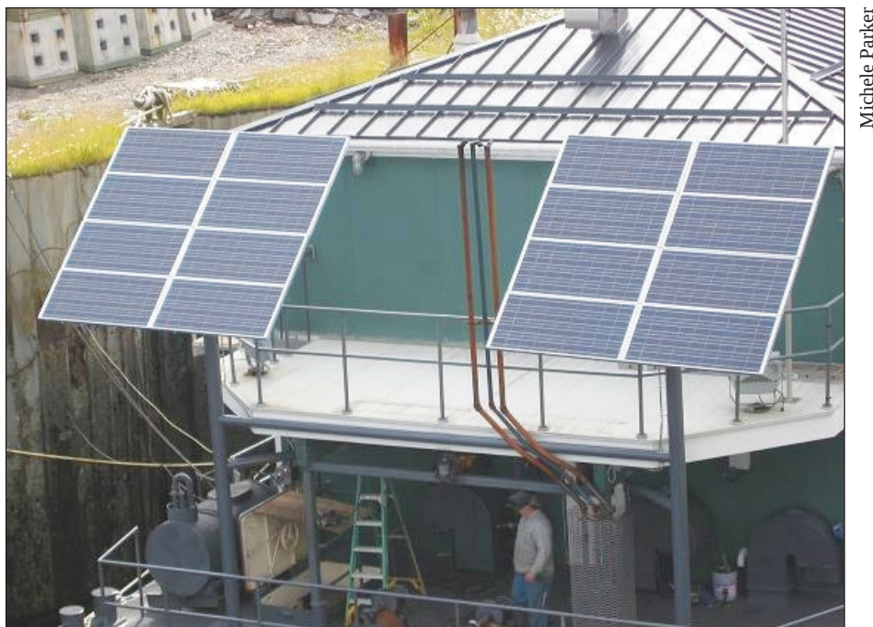
Figure 7—In 2011, the Tongass National Forest equipped its Steelhead Barge, which it uses as a floating bunkhouse, with solar arrays. The solar panels eliminate the use of 4,000 gallons (15,141 liters) of fuel oil a year, saving $60,000 and reducing greenhouse gas emissions.
