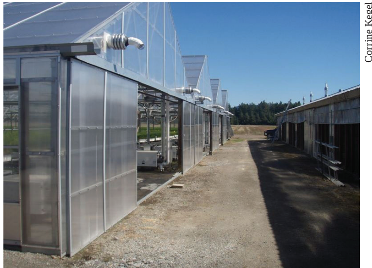
Figure 2—Forest Service nursery at Coeur D’Alene, Idaho Panhandle National Forest. By modernizing refrigeration, lighting, and heating, ventilation, and cooling systems, the nursery cut energy usage by 80 percent.
