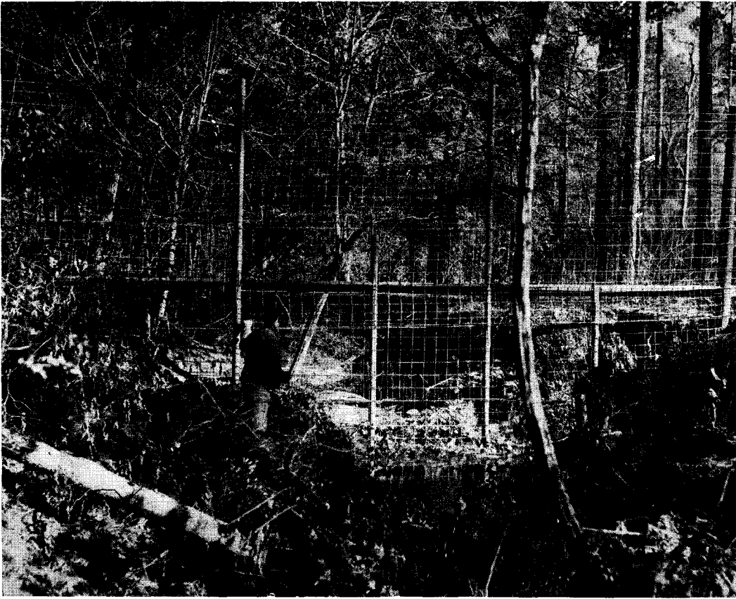
Fig. 2. A 9-foot deer-proof fence across a channel 25 feet wide. The installation has withstood floodwaters up to the horizontal beam.
