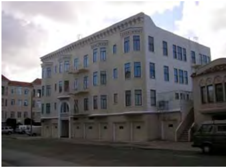
Figure 1. Example of a soft-story woodframe building in California (Photo credit: M. Gershfeld)
