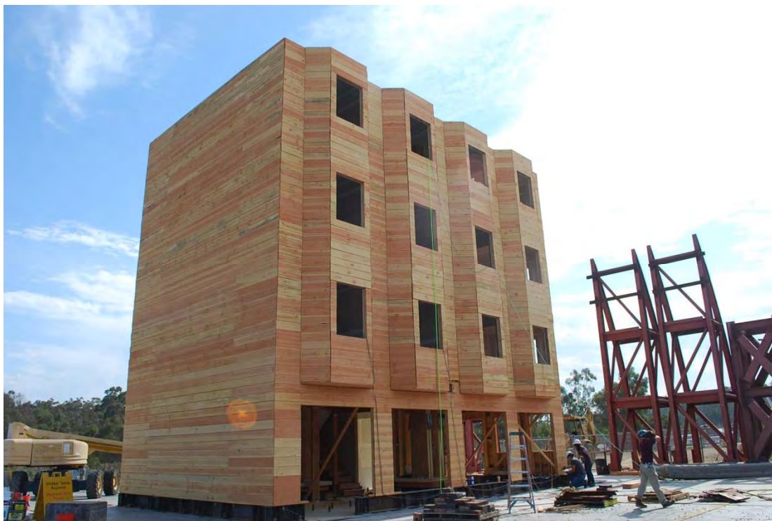
Figure 5. Four story shake table test building at NEES@UCSD
