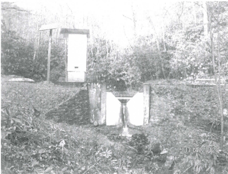
Figure 3.1 Upstream view of 90° V-notch weir installation on WS 7, November 2012. (USDA Forest Service photo)
