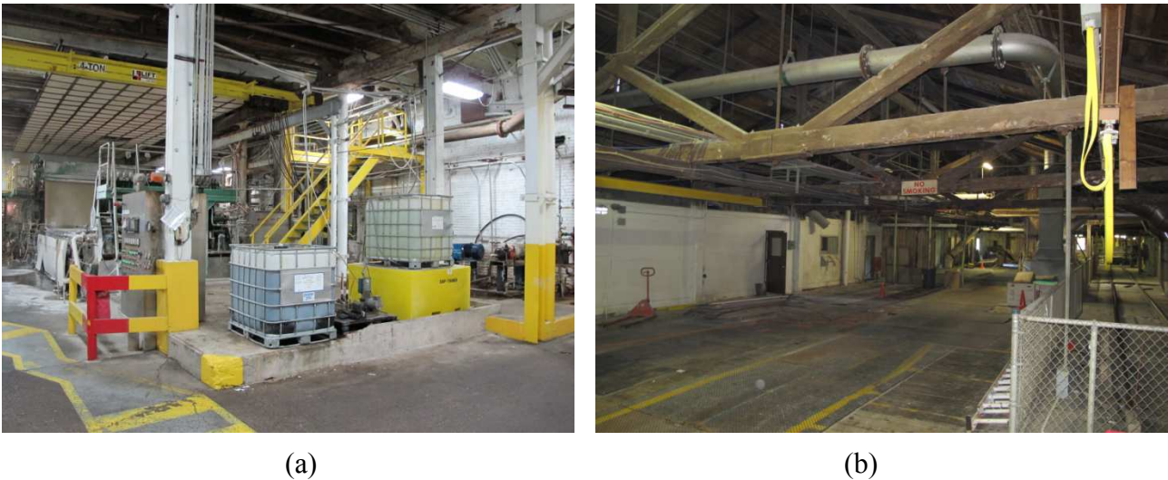
Figure 1. Heavy timber structures of a century-old industrial building. (a) Interior view of the first floor in the building showing a paper machine operation; (b) Interior view of the second floor in the building showing roof trusses and the floor.
