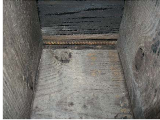
b. Tension rod between girder and deck
