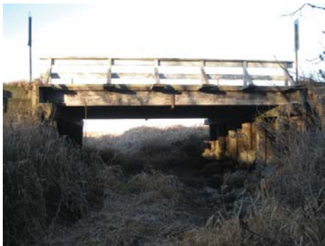
Fig. 2 Timber girder bridge elevation view from Cluster 1 in Bremer County
