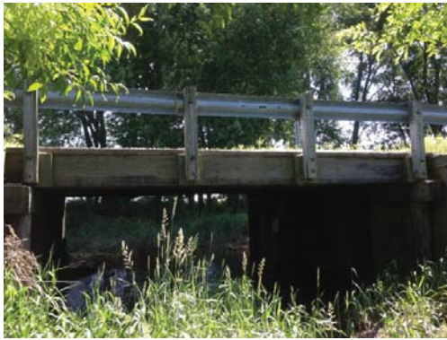
Fig. 4 Timber girder bridge elevation view from Cluster 2 in Blackhawk County
