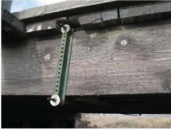
a. Exterior tension rod connection
