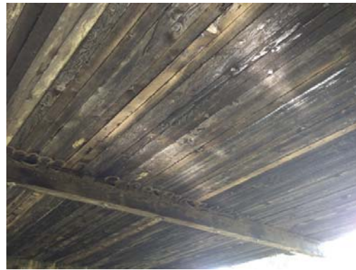
Fig. 7 Timber deck bridge underside view from Cluster 3 in Clarke County
