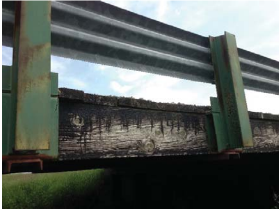
Fig. 10 Bremer 2 guardrail detail
