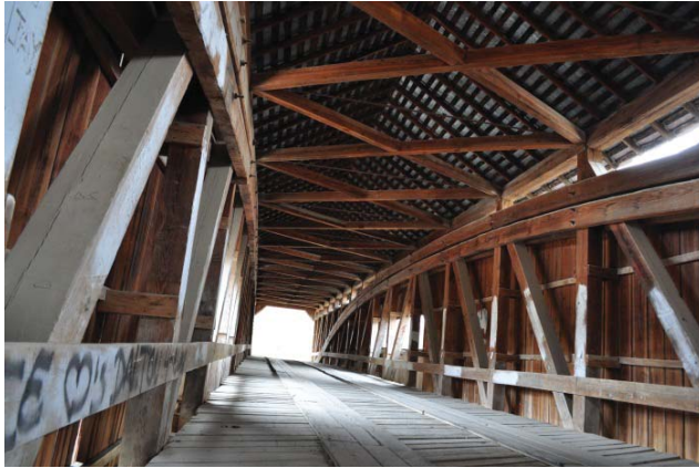
Fig. 1 Interior view of the Cox Ford Bridge showing the Burr arch truss configuration
