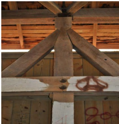
Fig. 11 Connection between V4 and the two diagonal members at the center span of the bridge
