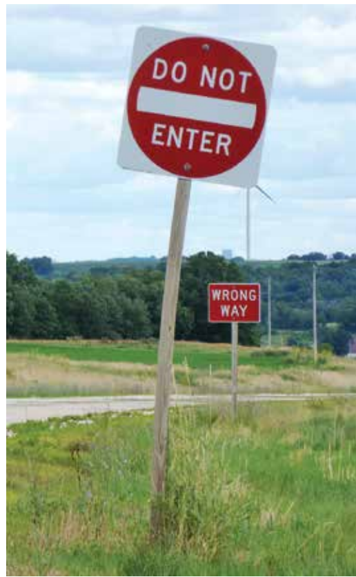
Figure 24. Warp appears to be more common, or at least more visible, in single-post than two-post signs.
