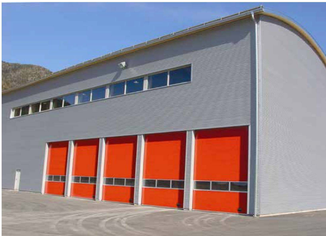
Figure 29 Kommissionshalle, Katsch, Austria (courtesy of KLH)
