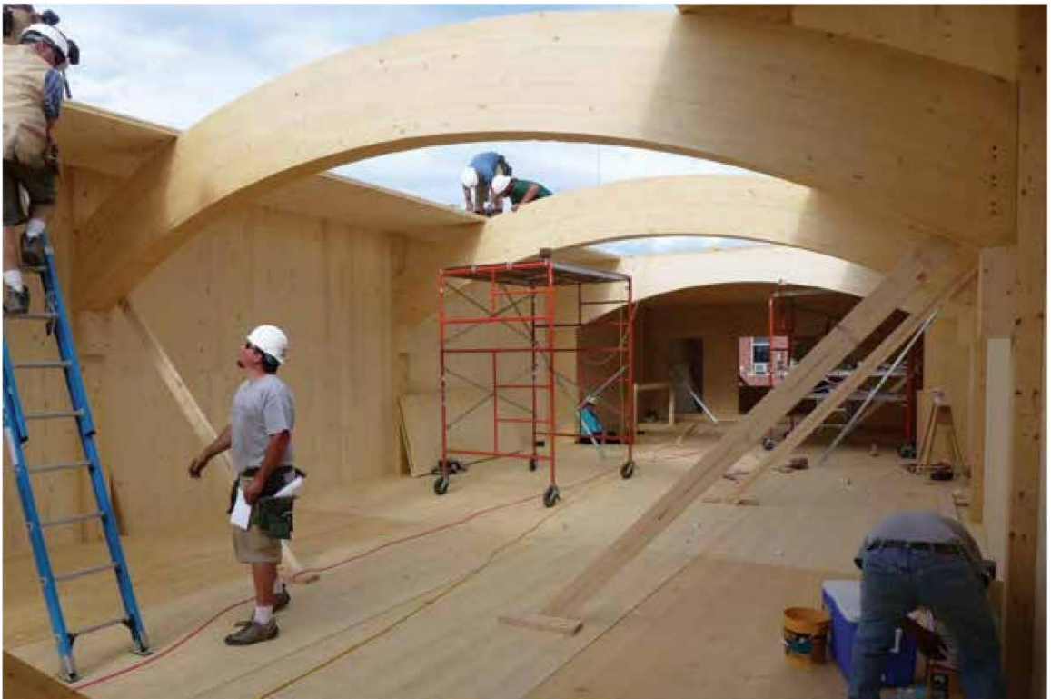
Figure 25 Montana Long Hall (courtesy of Structurlam Products Ltd.)
