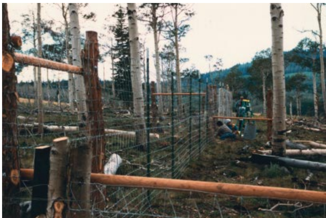
Figure 3 —The South Last Chance exclosure under construction in July 1996. The low fence to exclude domestic livestock is in the immediate foreground. The high fence to exclude all ungulates is in the background. Photo by Nate Yorgason.
