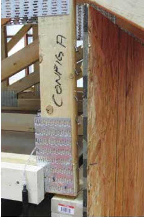
Figure 11. Primary failure mode of Test A.
