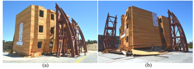
Figure 15: The test building following collapse: (a) front of building with garage openings not visible due to collapse; (b) back of the building
