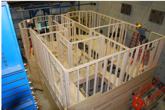
Figure 3: Physical substructure under construction at NEES-UB Laboratory.
