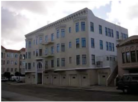
Figure 1. Example of a soft-story woodframe building in San Francisco, California (Photo: M. Gershfeld)
