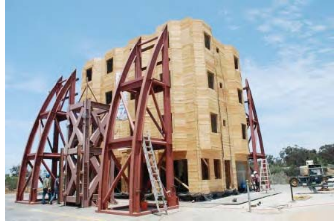
Figure 21. Structure with steel towers in place to prevent the building from hitting the control room should it collapse during testing
