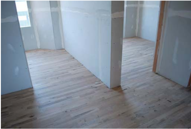
Figure 18. Interior view of completed structure (2 nd floor)
