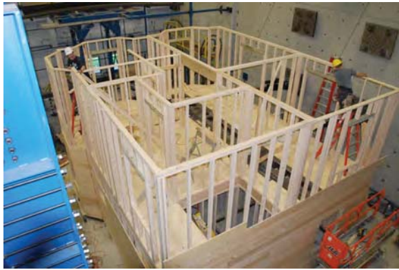
Figure 5. Third story framing nearing completion
