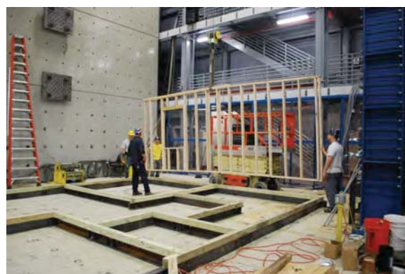
Figure 4. First wall being installed for the second story of the NEES-Soft test building
