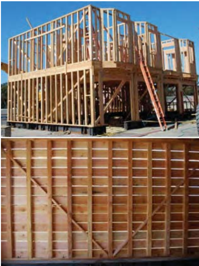
Figure 18. Exterior wall bridge bracing
