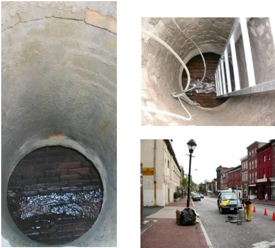
Figure 3. Baseflow in the Baltimore storm drain (left, top). Neighborhood around the manhole used for access for storm and baseflow sampling (K. Belt Photos).
