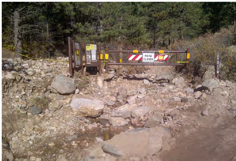
The flood caused severe damage to bridges and roads on the Arapaho and Roosevelt National Forests. (Image credit: top and bottom, Arapaho and Roosevelt National Forests)
