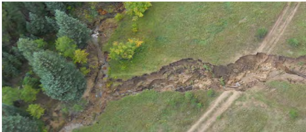
The flood caused major washouts and erosion on the Arapaho and Roosevelt National Forests and in surrounding communities. (Image credit: Arapaho and Roosevelt National Forests)
