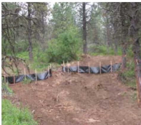
Silt fences installed on two skidder trails to measure soil erosion in the Payette National Forest, Idaho.
