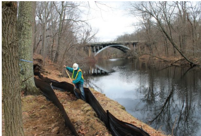
Figure 36. Silt fence installation prior to harvesting in a SMZ in Connecticut, USA (Photo courtesy of Newstimes).
