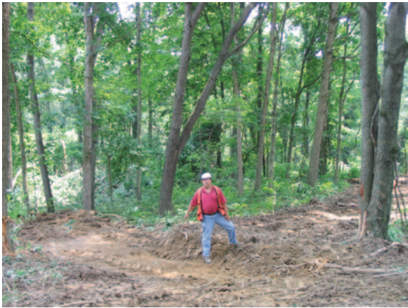
Fig. 16.6 Water bar constructed on a modern skid trail following guidelines developed in the Fernow Experimental Forest in the 1950s. (Source: http://www.muskingumtrees.com/water-bar.jpg )
