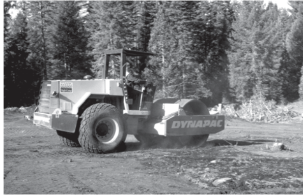
Fig. 23.9 Achieving uniform soil compaction at Challenge through perpendicular passes of a vibrating roller
