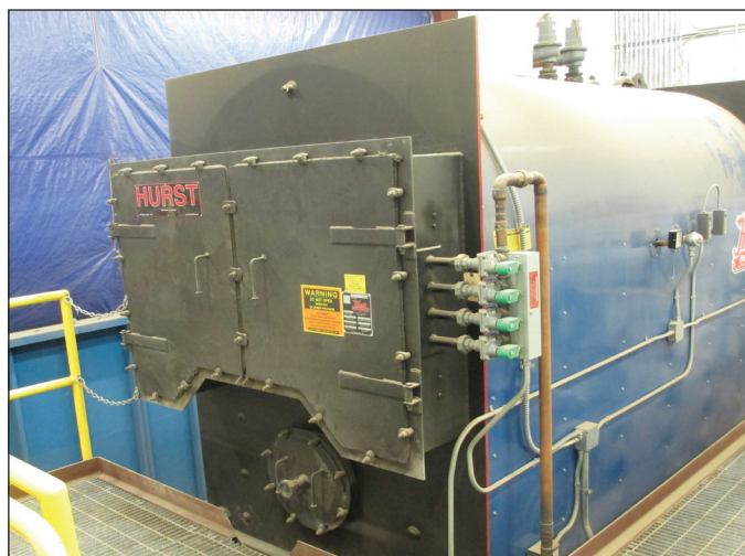
The wood chip boiler at Delta Junction School, Alaska.
