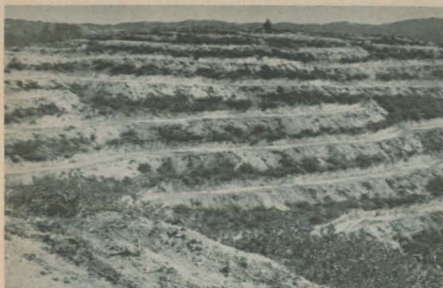
Figure 1. Typical example of the steep slope terracing done on 15,000 acres of Boise National Forest.
