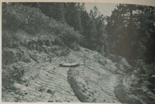
Figure 2. Sloped terrace showing track berms. Furrows formed by berms are preferred planting spots.
