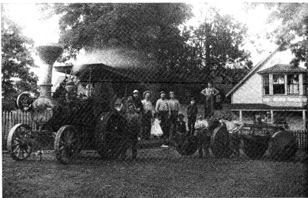
Road engine and empty log truck on the south side of the Leach residence at Challenge in 1892.
