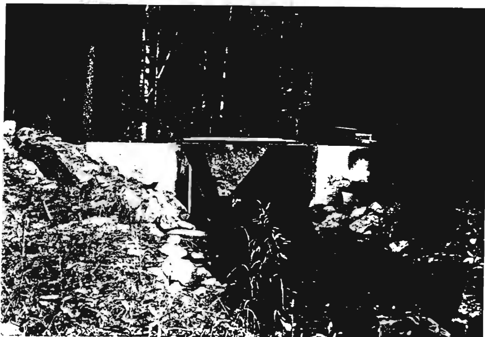
Figure 11--Photograph of 3-1/2-foot H-flume on Bubbling Creek near mouth.
