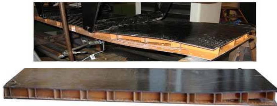
Figure 5. Interface shear failure [2].
