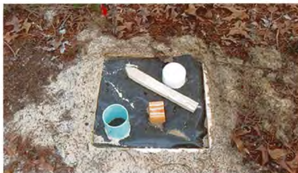
Fig. 3. A concrete slab plot after treatment before concrete pouring.
