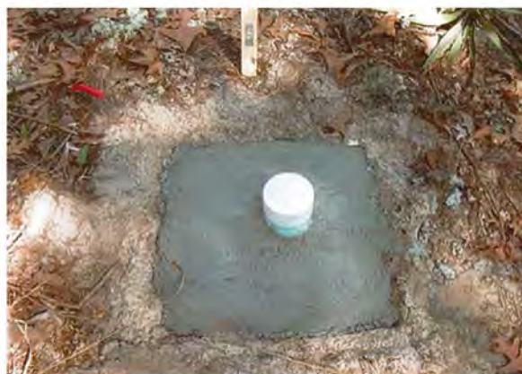
Fig. 4. A completed concrete slab plot.
