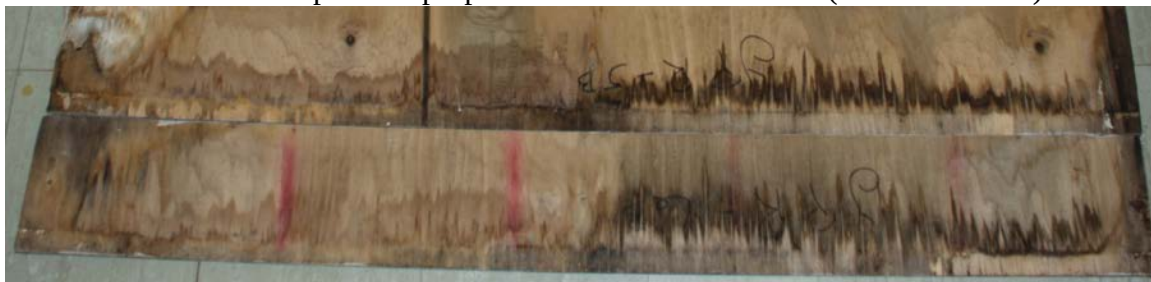
Fig 3: Back side of 2 panels after exposure, with caulked edges and no bottom gap showing water staining, more severe with the Venturi effect and gap behind boards (right) while end decay is more pronounced without gap behind boards (left).
