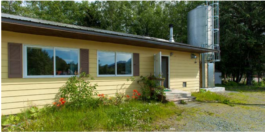
The silo on the side of the Senior Center (above) holds 12 tons of pellets—about a year's supply. Unfortunately, it is a bit too tall for many pellet delivery trucks.
