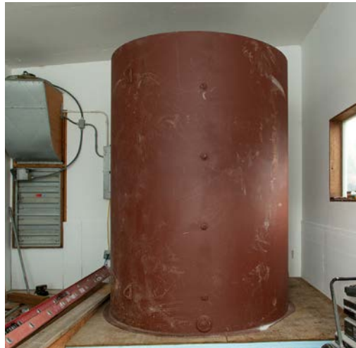
The biomass heat plant (upper left) houses the wood chip boiler (left) and hot water storage tank (below). Hot water is circulated through underground insulated tubing to several of the nearby buildings (above).
