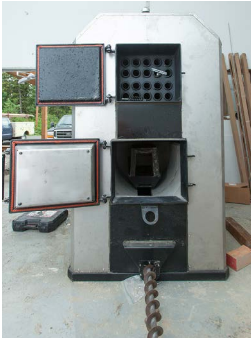
The biomass heat plant (upper left) houses the wood chip boiler (left) and hot water storage tank (below). Hot water is circulated through underground insulated tubing to several of the nearby buildings (above).
