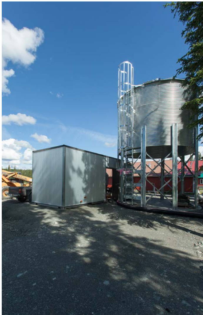
The containerized pellet boiler system (left) reduces onsite installation complexity and costs, so communities can focus on the things that matter—like this modern dental office (below).
