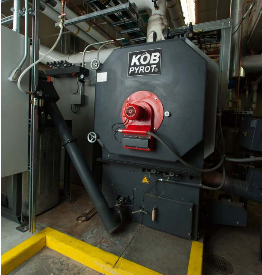
The Sealaska Building in downtown Juneau (upper right) is heated in large part by this fully automatic 750,000 Btu/hr KÖB/Viessmann pellet boiler (above). Wood pellets are delivered several times a month in bulk by this converted grain delivery truck (right).
