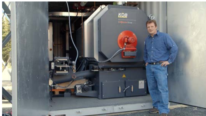
The containerized pellet boiler system (left) reduces onsite installation complexity and costs, so communities can focus on the things that matter—like this modern dental office (below).
