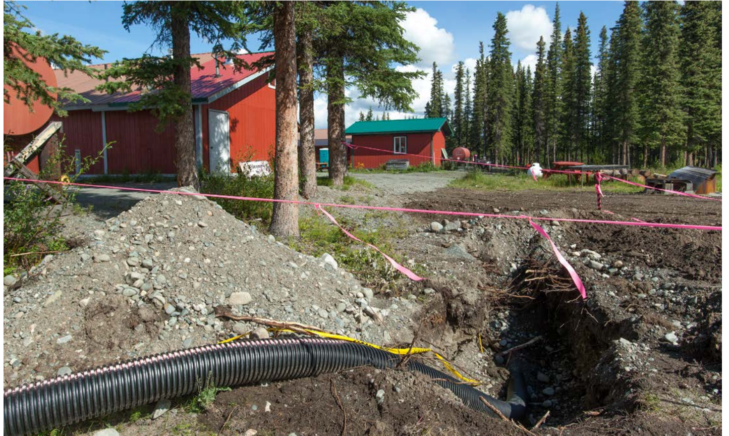
Heat from the pellet boiler (left) is delivered to the various buildings by circulating hot water through buried insulated piping (above).
