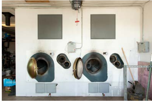
The tribal heat plant (right) houses two side-by-side GARN WHS 3200 cordwood boilers (above) capable of producing 700,000 Btu/hr each.
