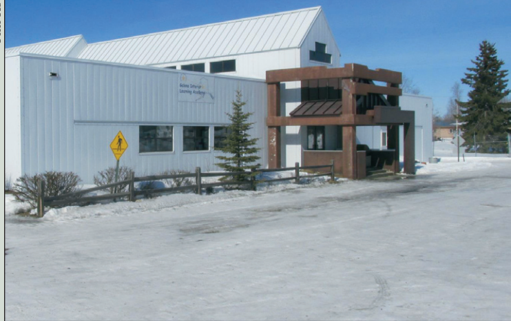
The Galena Interior Learning Academy in Galena, a remote rural village on the Yukon River. Over 100 high school students from 80 villages attend this boarding school. The school's inefficient diesel heating system is being replaced by a wood-fired boiler that will use wood chips sourced from regional tribal corporation land. The city of Galena, the local tribal council, and the school came together to pool resources and support this project.
