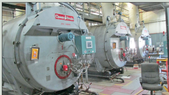
The diesel boilers that heated the Galena Interior Learning Academy once burned 1 million gallons of oil a year. This fuel had to be barged in, pumped into a pipeline, and stored, incurring transportation expense and the risk of environmental contamination.
