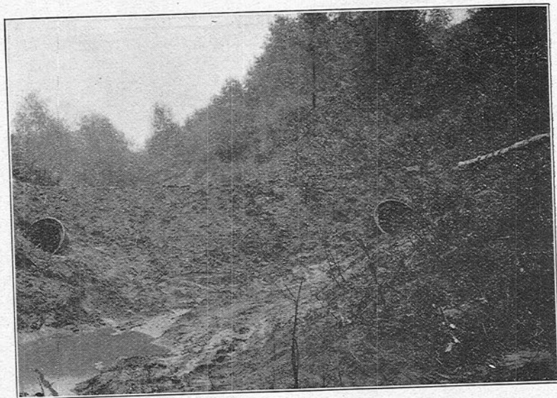
FIG. 43.—THE WISCONSIN TYPE OF EARTH FILL DAM
