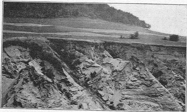
FIG. 19.—TERRACE SOILS READILY UNDERMINED
