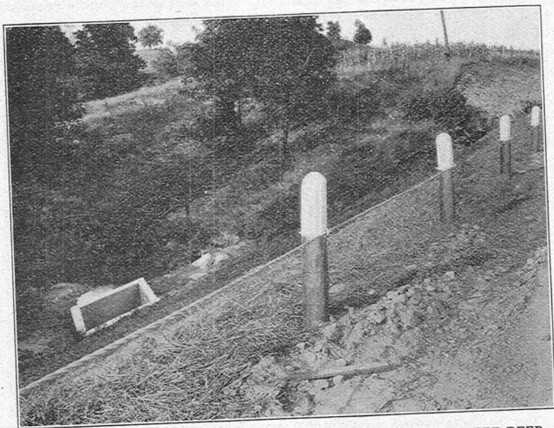
FIG. 46.—A HIGHWAY CULVERT WITH A DROP-INLET FIFTEEN FEET DEEP This serves exactly the same purpose as a soil-saving dam and is very worth-while to the adjacent land-owner since the gulch has filled in the few months since this was completed.
